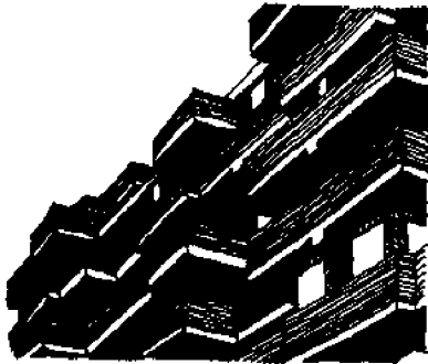
Lillington Gardens housing in Westminster, by Darbourne and Darke, in which modern architecture is combined with 'traditional' materials
